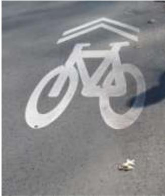
Shared lane markings (“sharrows”) indicate where cyclists should ride in a shared travel lane to be safe from opening doors on parked cars or other hazards. Motorists drive as normal in a shared lane when no cyclists are present; when cyclists are present, motorists should slow down and pass with care, at a safe distance, and only when it can be done without endangering the cyclist or oncoming traffic.
